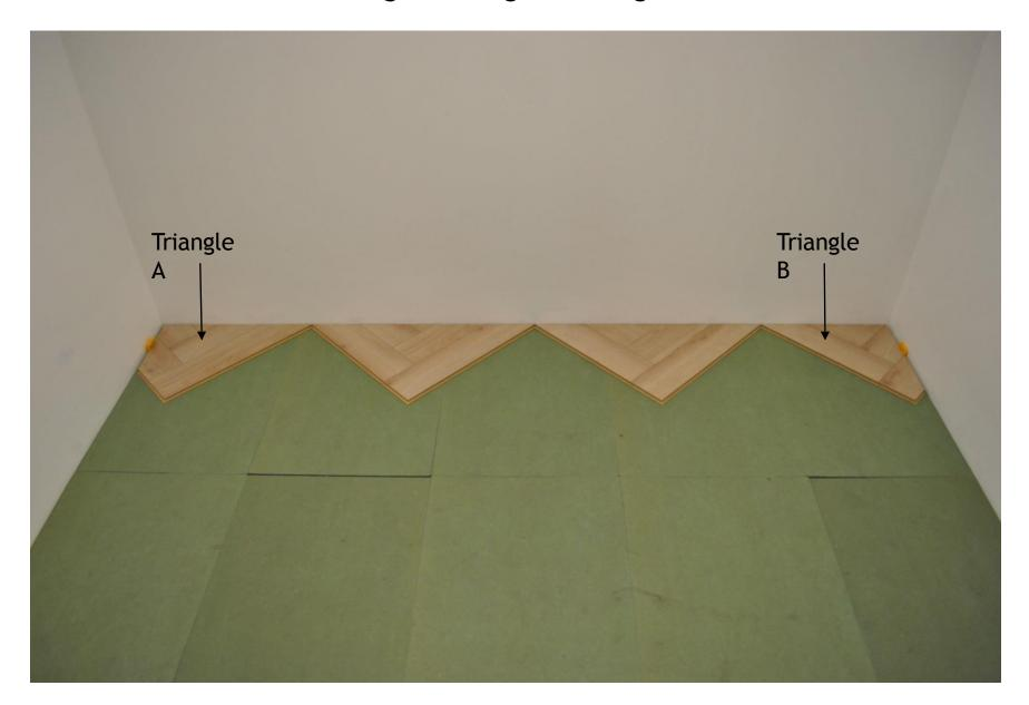
Install the first Left Planks (marked "Gauche" = G) with the Black Plastic tongue pointing to the left
