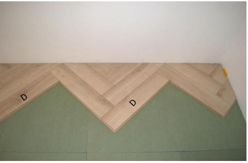
Measure the missing Right Plank piece D1
