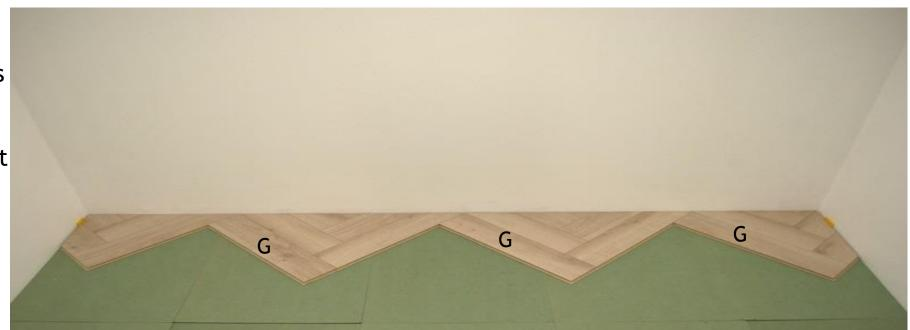
Next install the missing Left Plank piece G1
